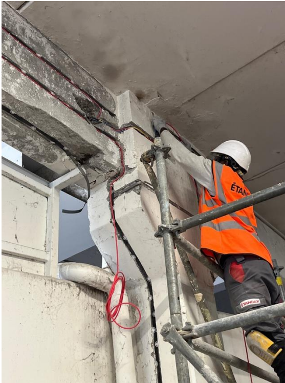
Installation of anodic cables (red) and cathodic cables (black) in the cutting grooves or at the surface of the facing
