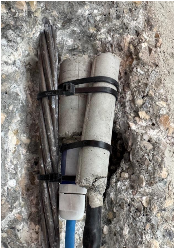
Installation of the pre-embedded sensors
