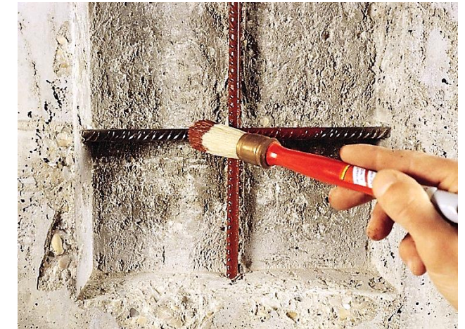
Application of a passivating primer on the rebars
