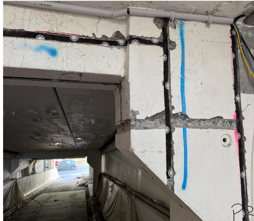
Ribbon installation in the cutting grooves
