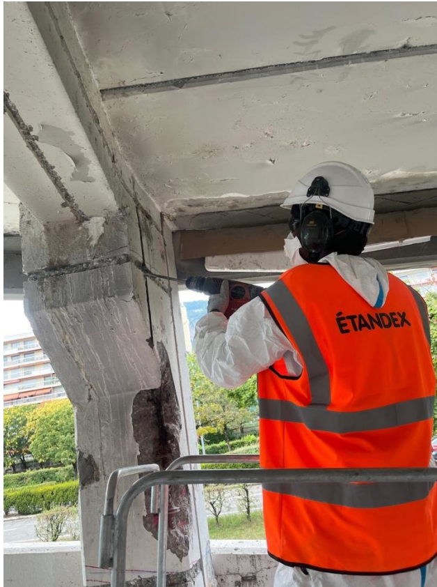
Cutting grooves in the various structural elements
