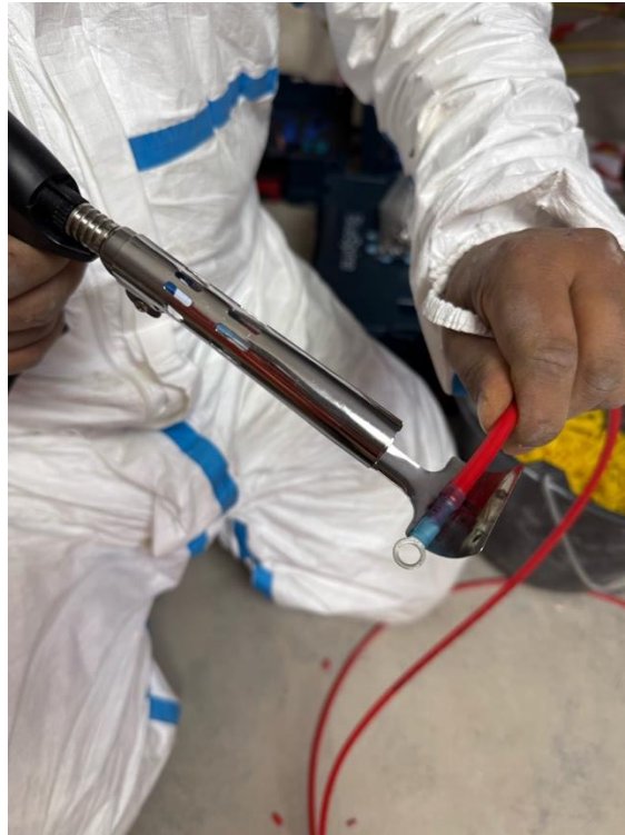
Anodic connections (+) with titanium connectors
