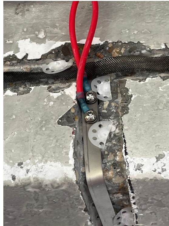
Anodic connections (+) with titanium connectors
