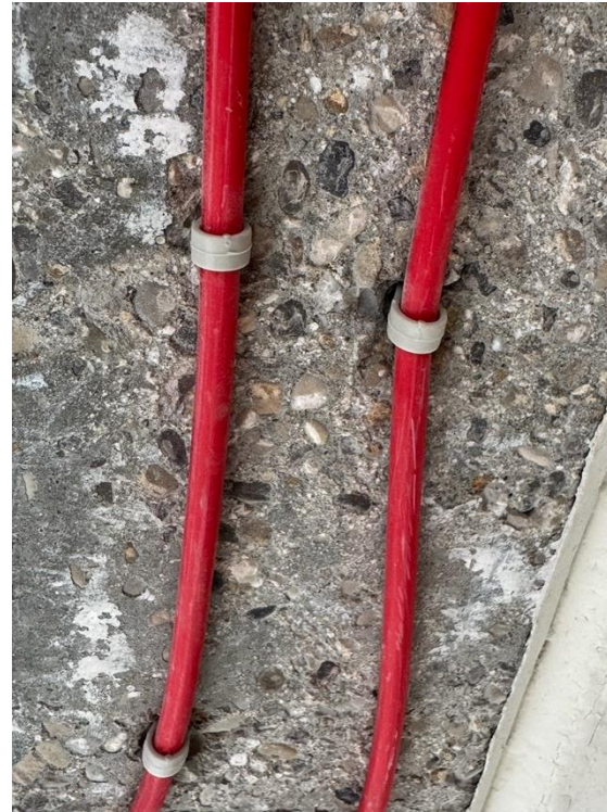
Installation of anodic cables (red) and cathodic cables (black) in the cutting grooves or at the surface of the facing
