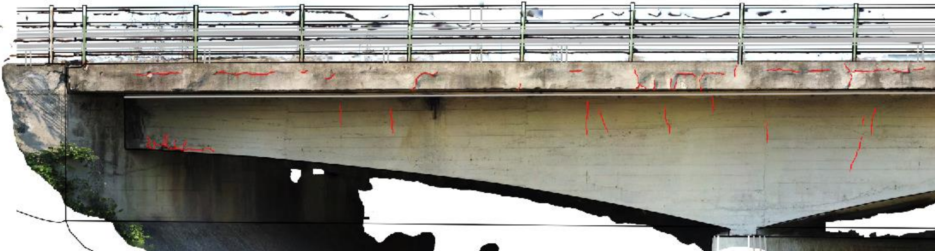
Reconstruction of the cracking pattern
